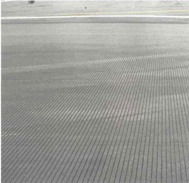
Grooves cut in the Logan Airport pavement in 2004
